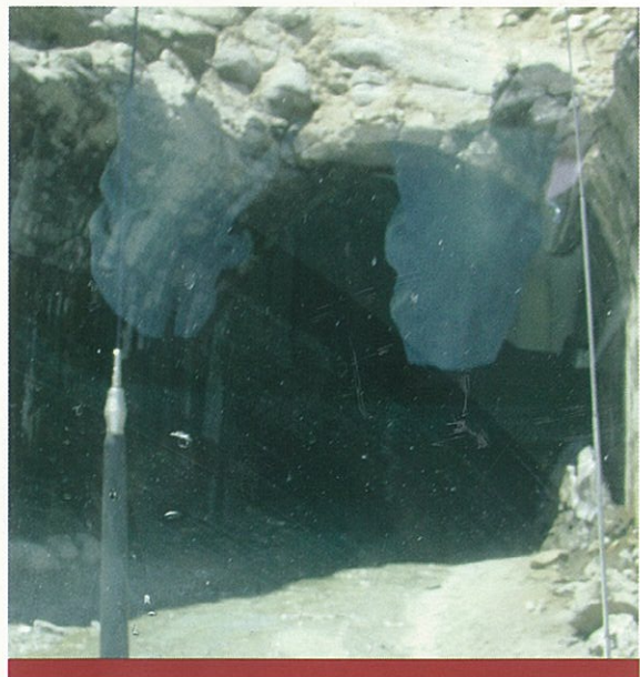
Figure 3. The highest tunnel in the world, Salang Tunnel, Hindu Kush mountains, Afghanistan, 2003. (The road and tunnel have since been substantially improved).
